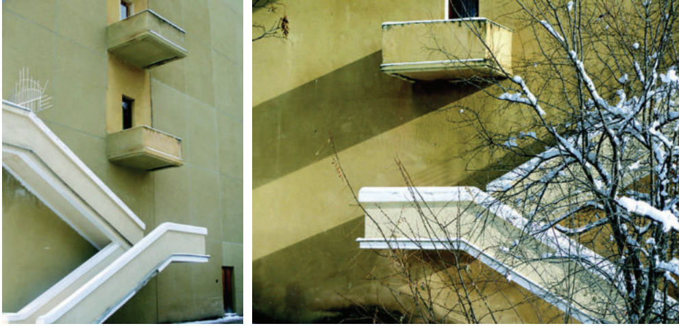
Fig. 40 Side Walls of the Western Wing. (Photo Udovicki)
