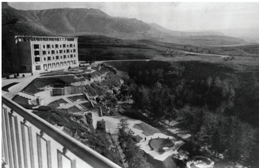
Fig. 2 General view of the East Wing of the “Ordžonikidze” Sanatorium in Kislovodsk, Caucasus, by M. Ginzburg, with Monumental Stairs by I. Leonidov in 1938. (Photo MuAr)
