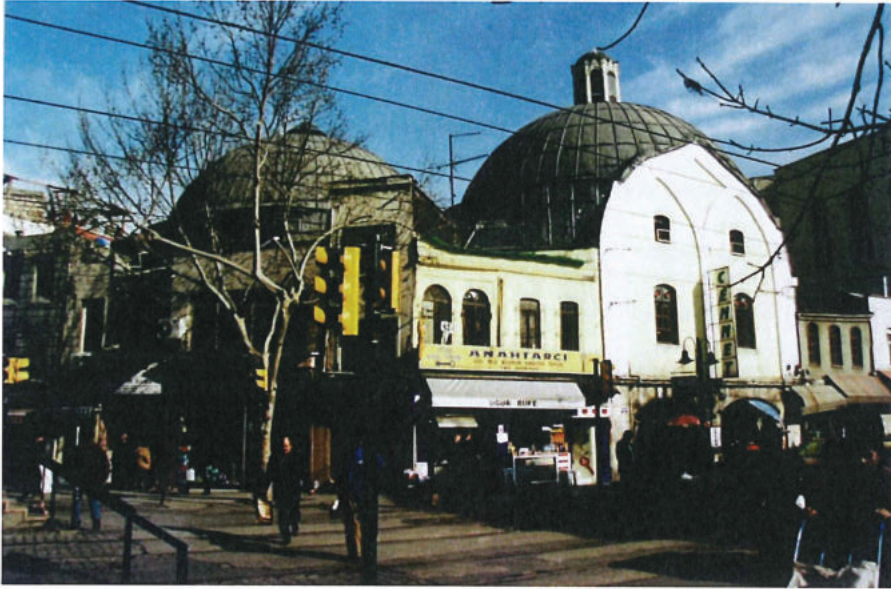
Fig. 3: Exterior of the Çemberlitaş Hamam. Source: Author's photograph.
